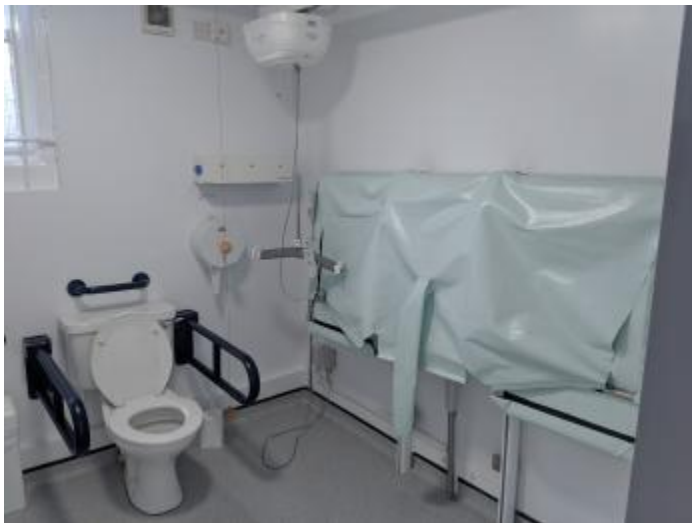
Accessible toilet and Changing Places facility.
