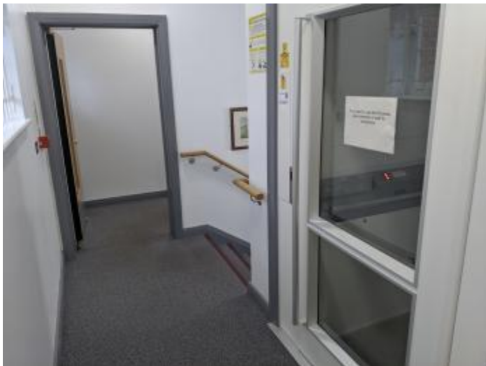
The lift on the first floor, near the stairs and door to the Community Room.
