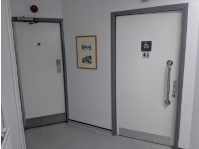
Doors to men's, women's and accessible toilets including a Changing Places facility.
